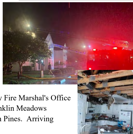
Figure 5-7: Eight Unit Two Story Building Fire Caused by Lightning
