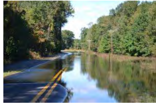
Flooding on Purnell Crossing Rd outside Berlin.
