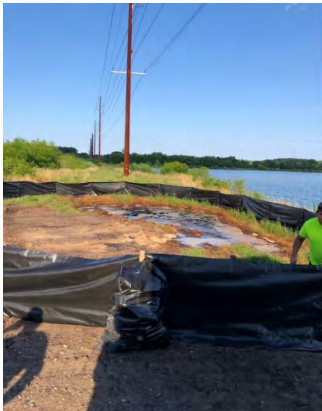
Photo submitted by Thom Gulyas. A "caustic chemical" spill with a pH level of 13 was discovered last Wednesday at Berlin Falls Park at the site off Old Ocean City Boulevard.
