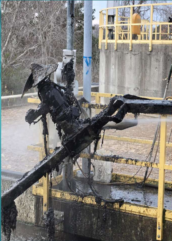
Mixer Guide Rail In Treatment Unit at Ocean Pines
