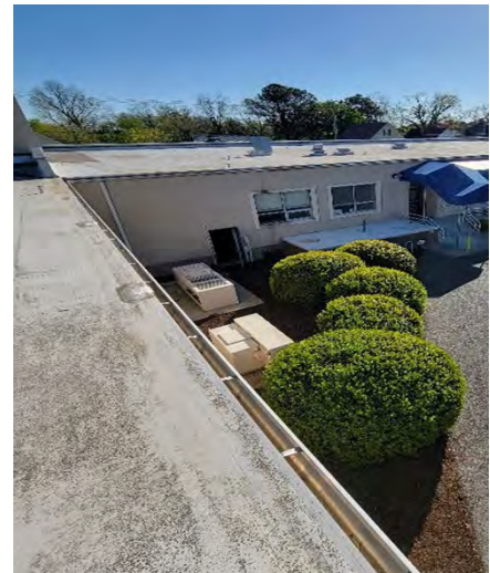
Rooftop Drainage Gutters
