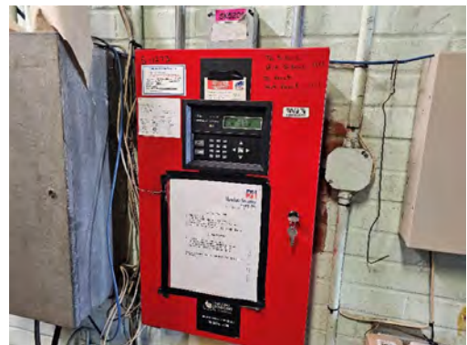
(EP19) Fire Alarm Control Panel
