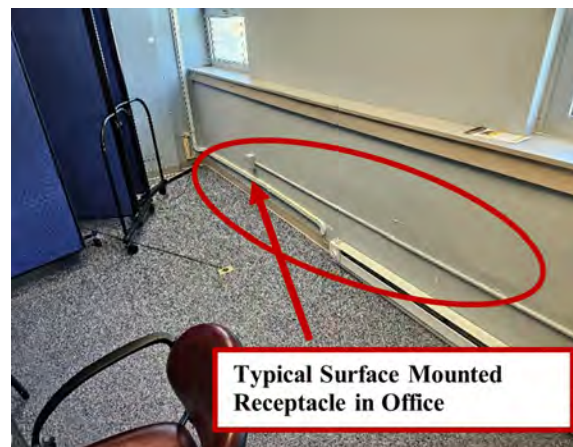
(EP7) Typical Surface Mounted Receptacle in Office
