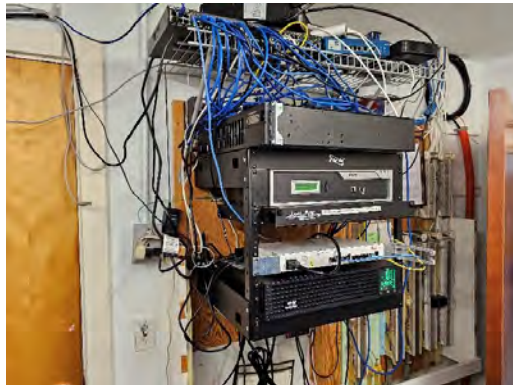
(EP26) & (EP27) Demarcation Equipment
