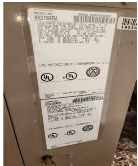
(MP11) York Condensing Unit Nameplate
