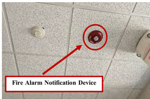
(EP21) Fire Alarm Horn/Strobe
