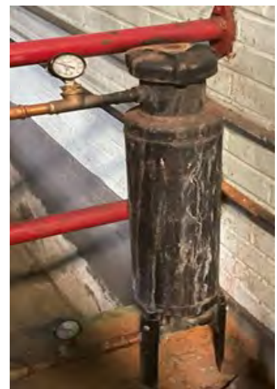
(MP4) Chemical Feed Tank
