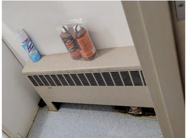
(MP15) Cabinet Unit Heater (typ.)
