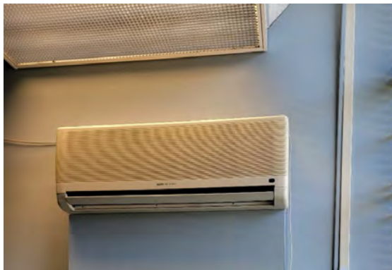
(MP14) Indoor Ductless System
