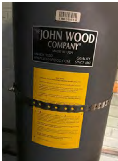
(MP3) Heating Water Expansion Tank
