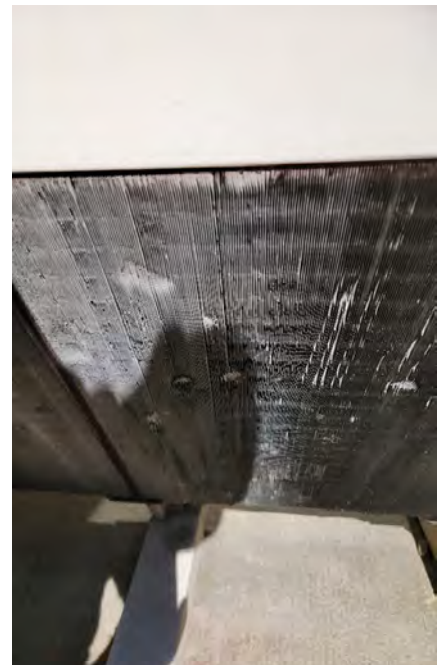
(MP10) Trane Unit Damaged Fins
