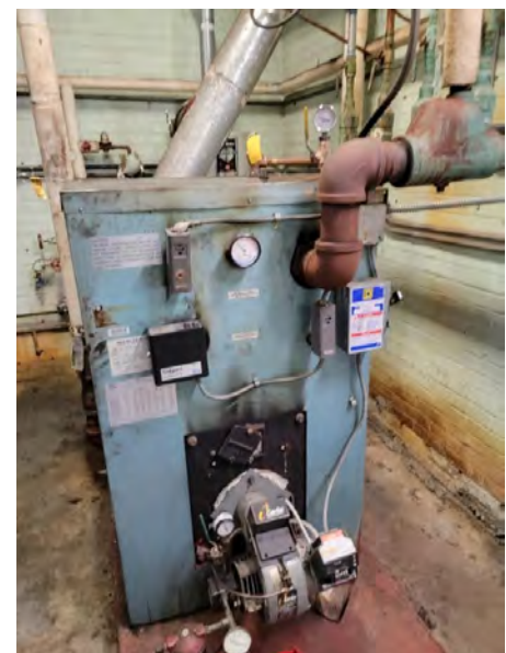
(MP2) Cast Iron Sectional Boiler
