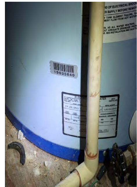
(MP19) Electric Water Heater
