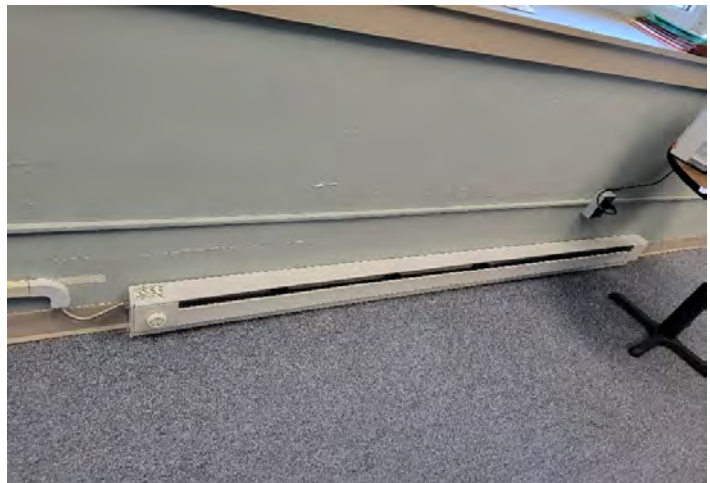
(MP16) Electric Finned Tube Radiator
