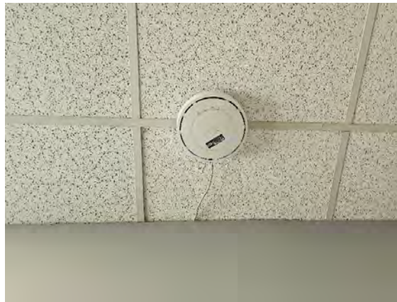
(EP28) Wireless Access Point
