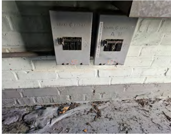
(EP8) Typical Disconnect Switch
