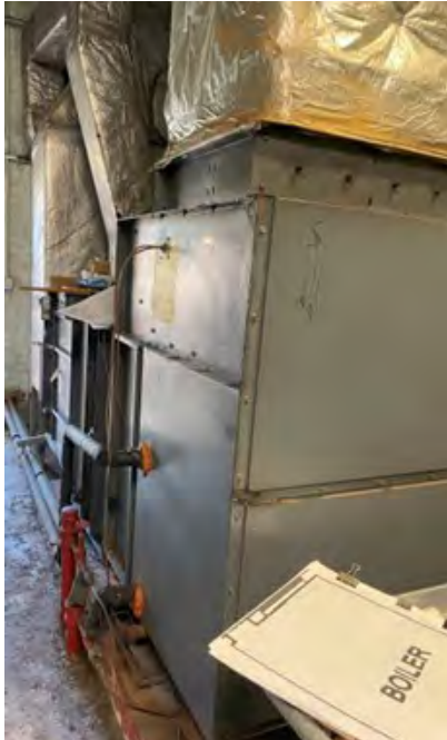
(MP7) Multi-Zone Air Handling Unit
