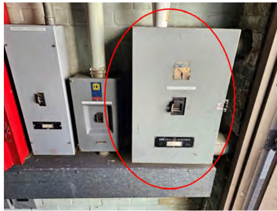
(EP2) 600A Enclosed Circuit Breaker
