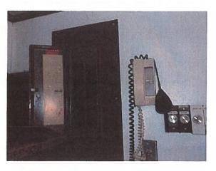
**208/120 VOLT SYSTEM** - single 100 amp three phase system with a household type circuit breaker boxes, which is not ignition protected. The generators have their own breaker panels. The wiring does not comply with ABYC standard E-11. I have noted the following:
