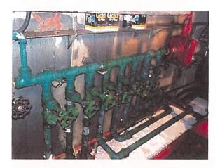
**FIRE PROTECTION:** the vessel is equipped with two electric pumps with fire hoses. There are carbon dioxide extinguishers and dry chemical fire extinguishers installed throughout the vessel. The fire extinguishers were being inspected at time of my inspection. The carbon dioxide extinguishers were not inspected at time of my inspection. An axe is mounted in the stairway to the pilot house. There are no smoke or carbon monoxide detectors installed.
