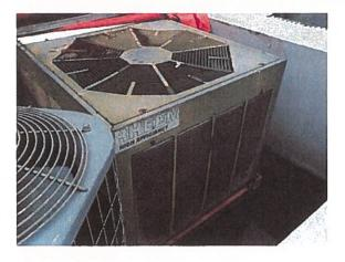
The vessel is also equipped with a Carrier camper style air conditioner in the ceiling in the pilot house, which does not work well. The air grid on the front section is missing.
