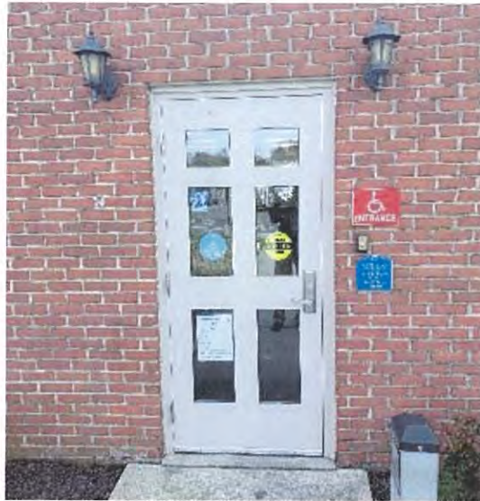
Photograph #16 – Wall Mounted Decorative Light Fixture
