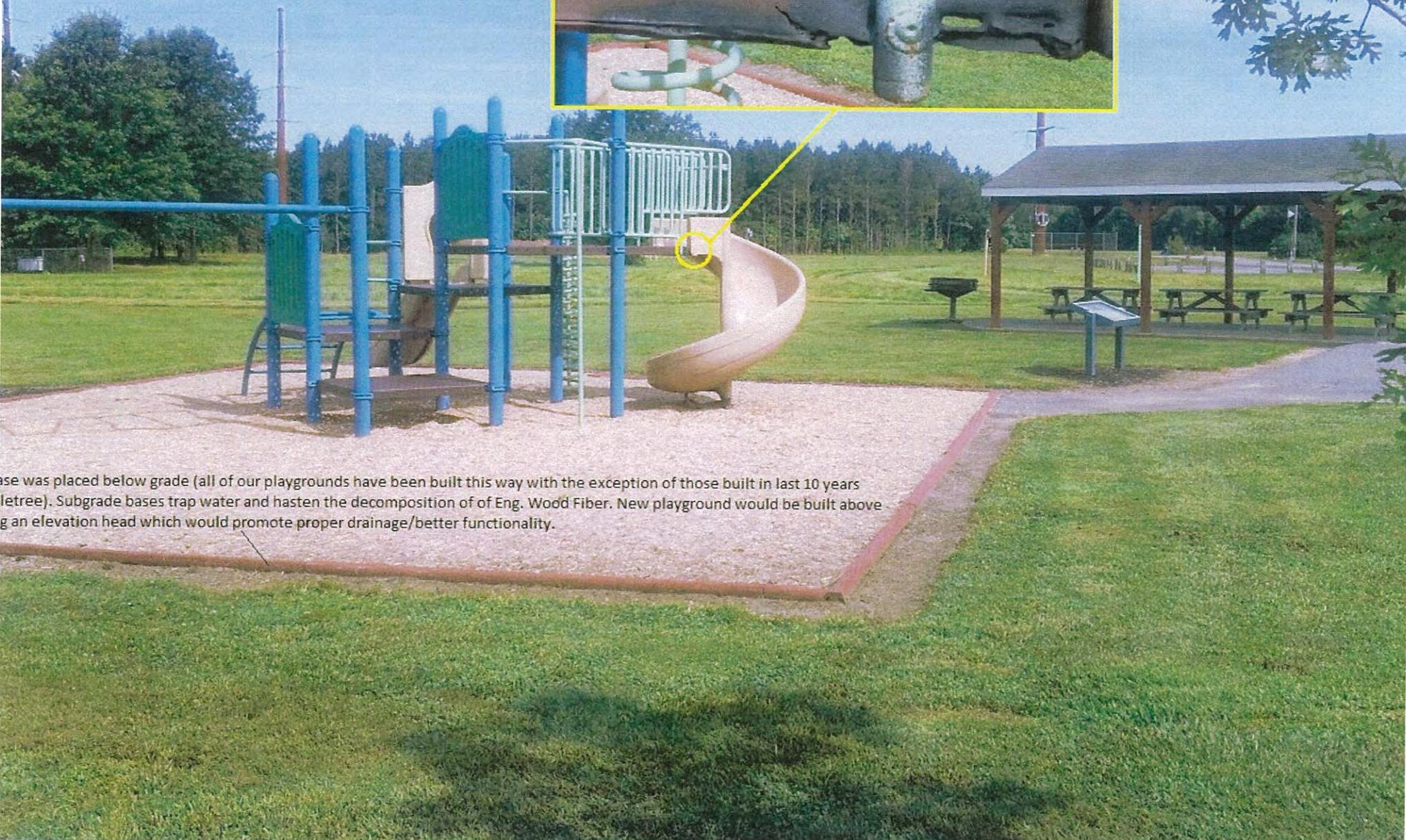
use was placed below grade (all of our playgrounds have been built this way with the exception of those built in last 10 years (retire)). Subgrade bases trap water and hasten the decomposition of of Eng. Wood Fiber. New playground would be built above an elevation head which would promote proper drainage/better functionality.
