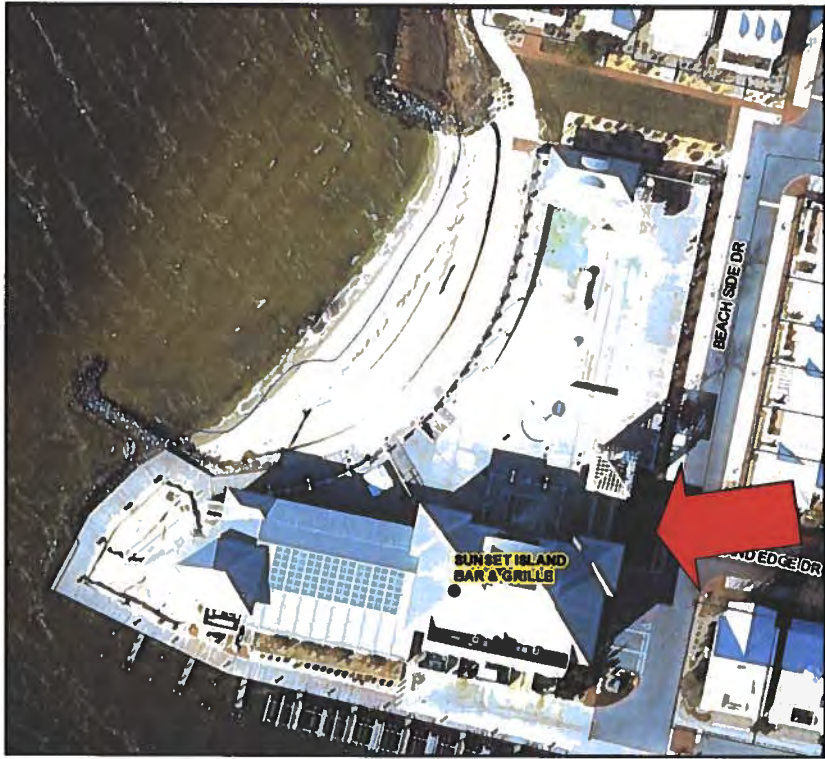
Pictures taken by: Harold "Skip" Cook, Board Investigator on April 15, 2020 Department of Development Review & Permitting—Technical Services Division—April 2020
