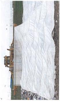
Speed and Productivity Deployment and retrieval of Tarpomatic tarps is significantly faster and more efficient than any other method of daily cover. In fact, on average, it takes approximately 15 minutes to deploy Tarpomatic tarps across a working face.
