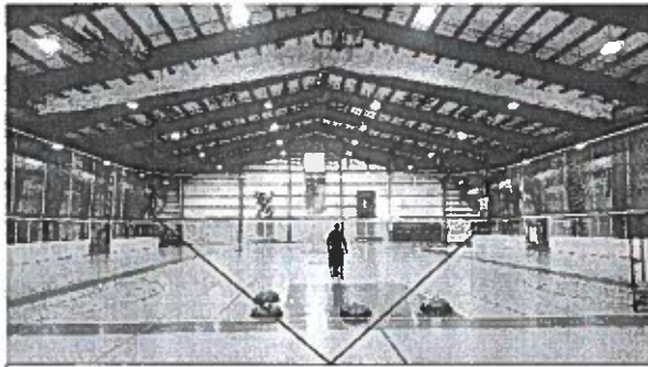
Photograph #4 – Non-Metallic Duct System with Blue DuctSox
