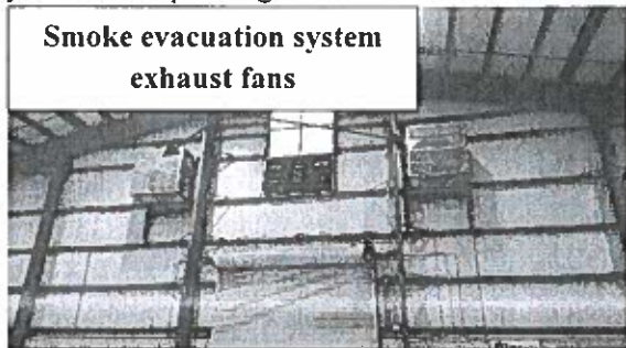
Photograph #6 – Smoke Evacuation System Exhaust Fans
