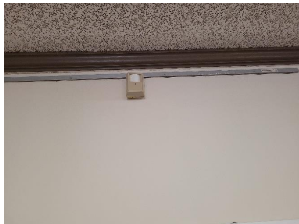
Photograph #56 – Motion Detector
