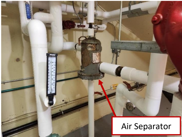
Photograph #7 – Heating System Air Separator
