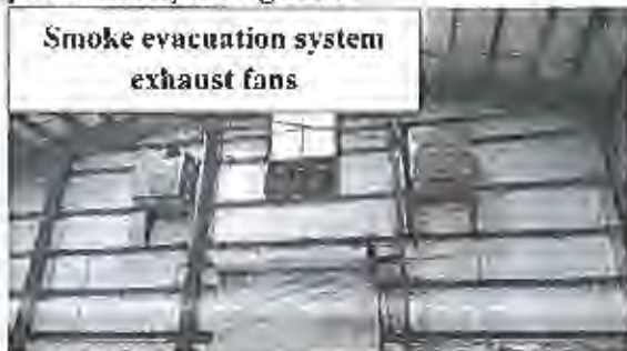
Photograph #6 – Smoke Evacuation System Exhaust Fans
