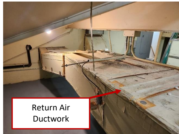
Photograph #26 – AHU #2 Main Return Air Ductwork
