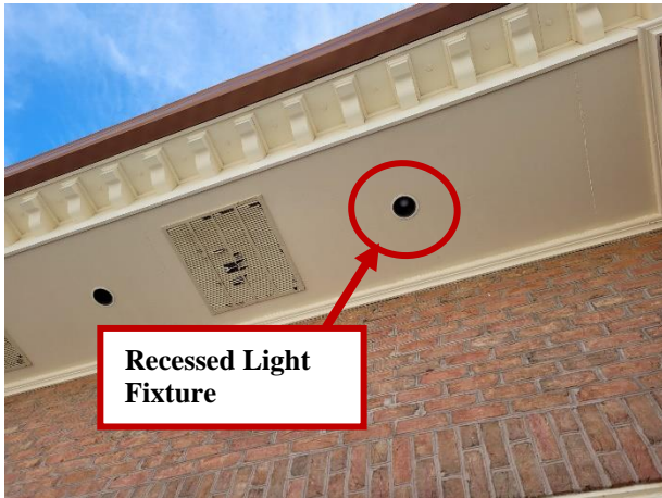
Photograph #48 – Recessed Light Fixture at exterior canopies
