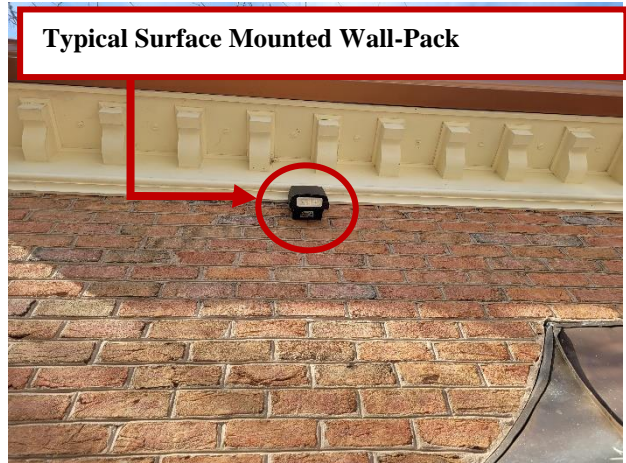
Photograph #49 – Typical Surface Mounted Wall-Pack
