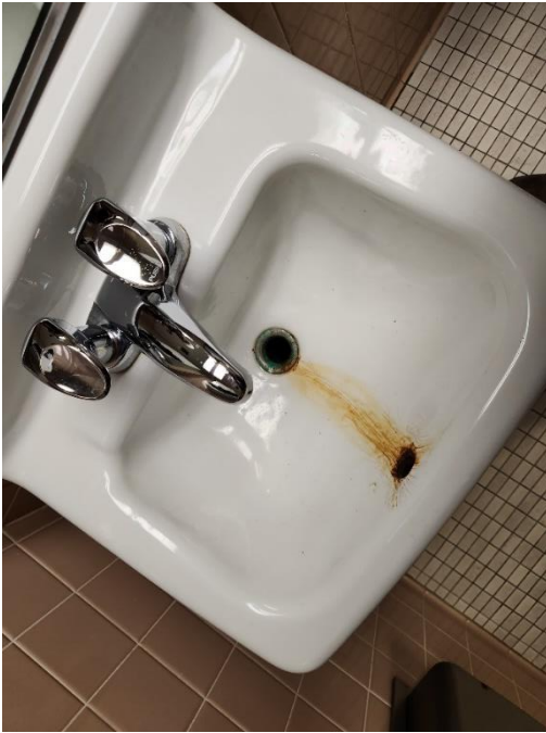
Photograph #29 – Typical Lavatory
