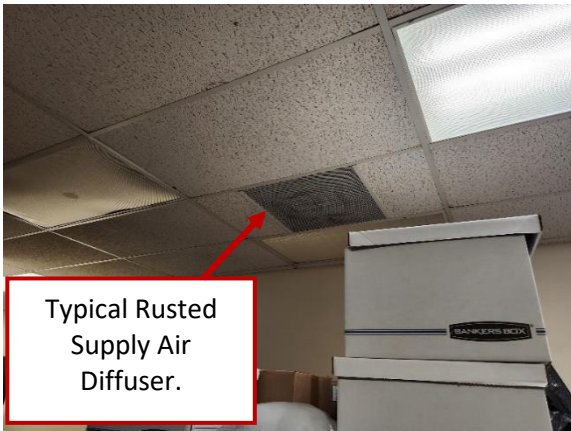
Photograph #25 – Typical Supply Air Diffuser
