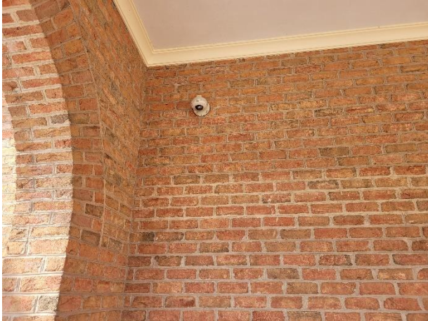
Photograph #57 – Exterior Video Surveillance Camera at Front Entrance
