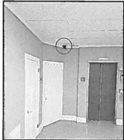
Photograph #21: Video Surveillance Camera
