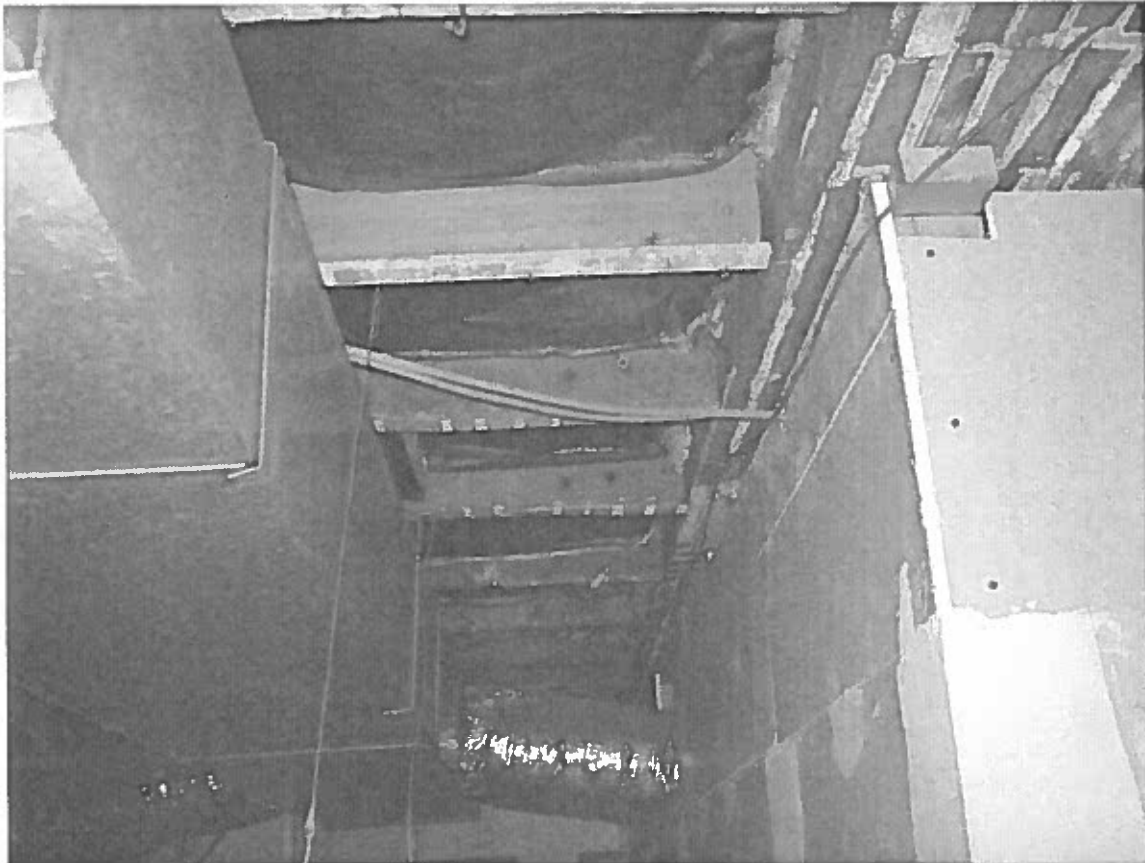
Photo 22 - Second floor framing 2 x 12 @ 16"
