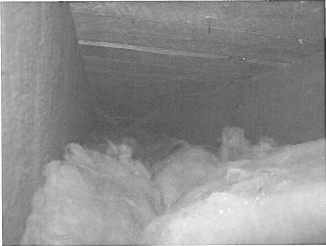
Photo 19 - Third floor framing 2 x 12 @ 16"
