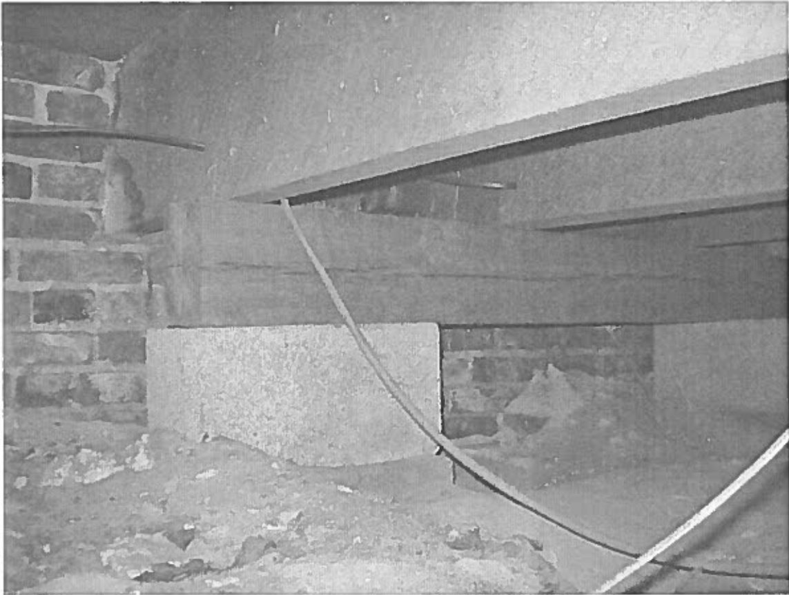
Photo 31 - - Supplemental supports at joist ends
