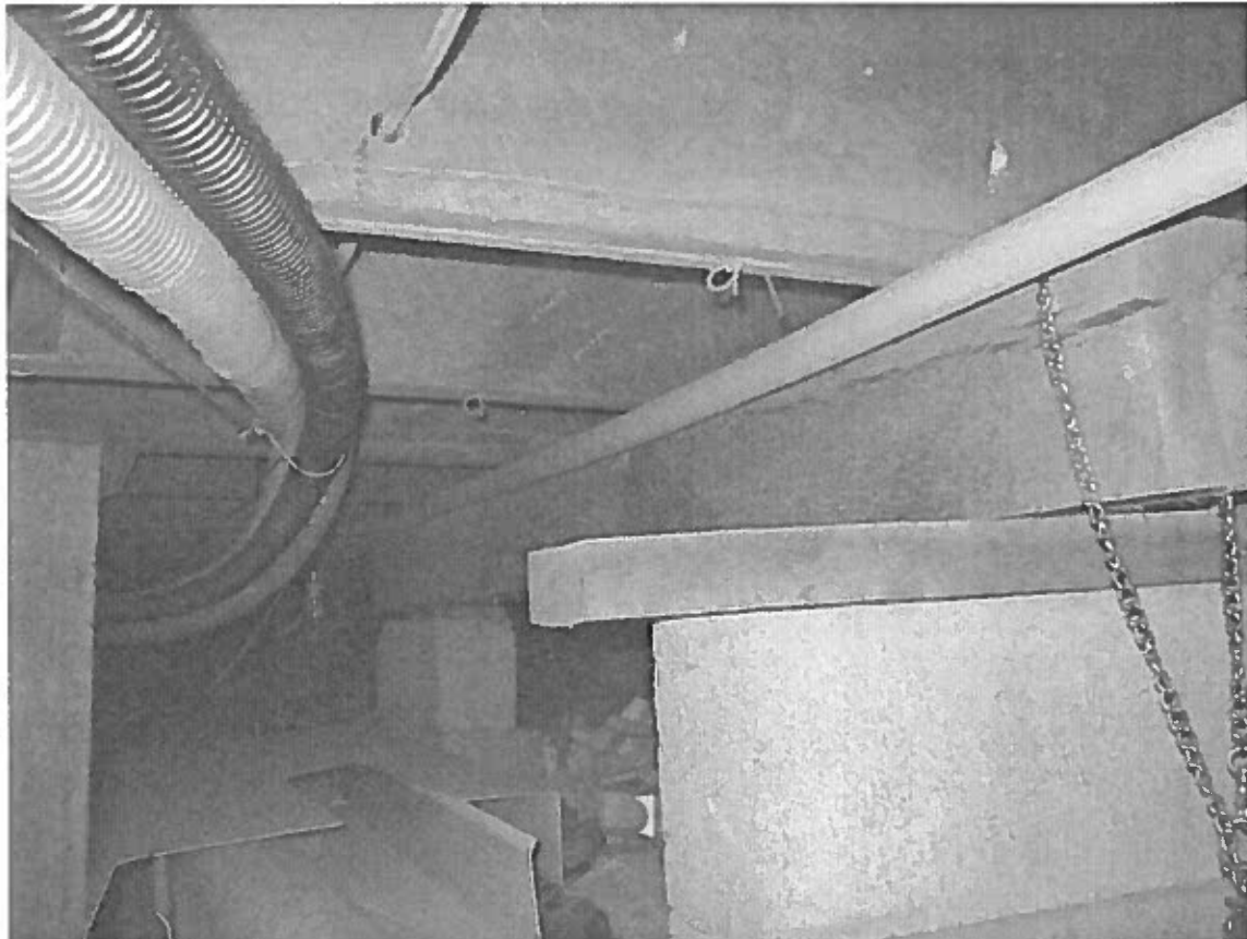
Photo 32 - Supplemental supports at joist ends
