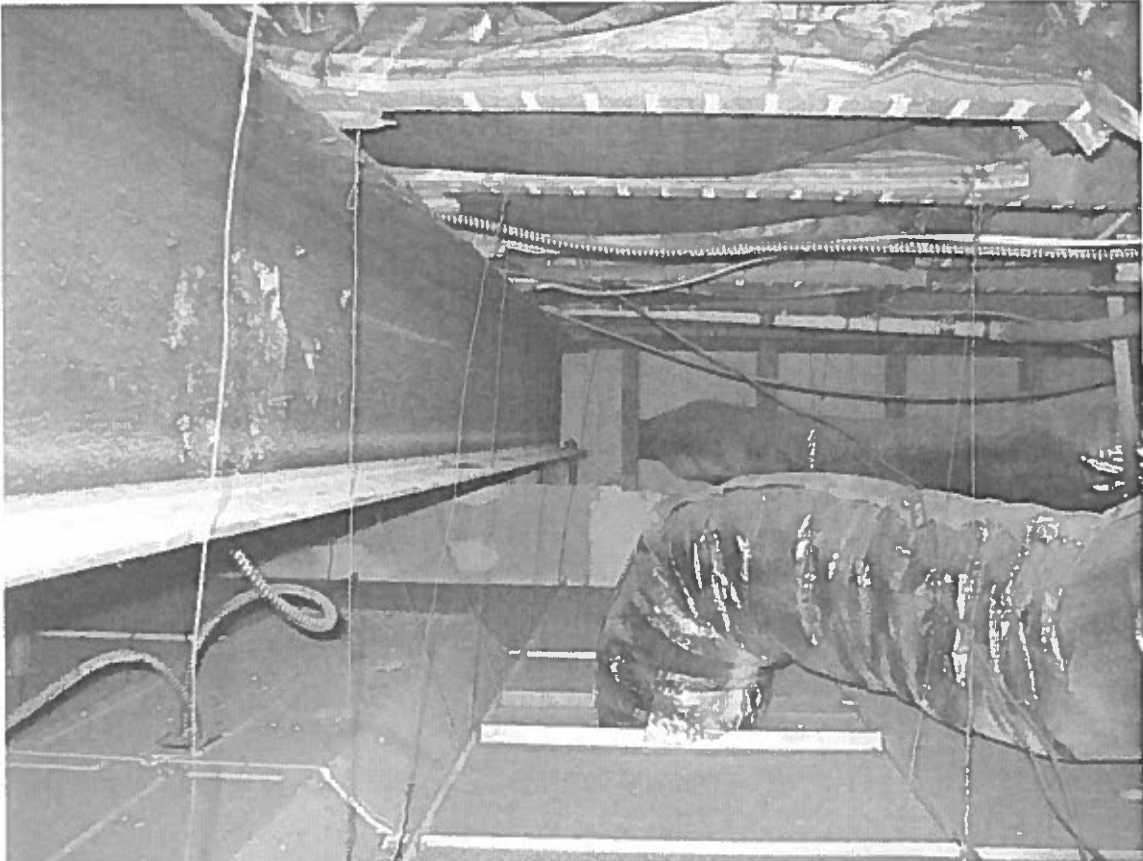
Photo 26- Supplemental support of second floor joists
