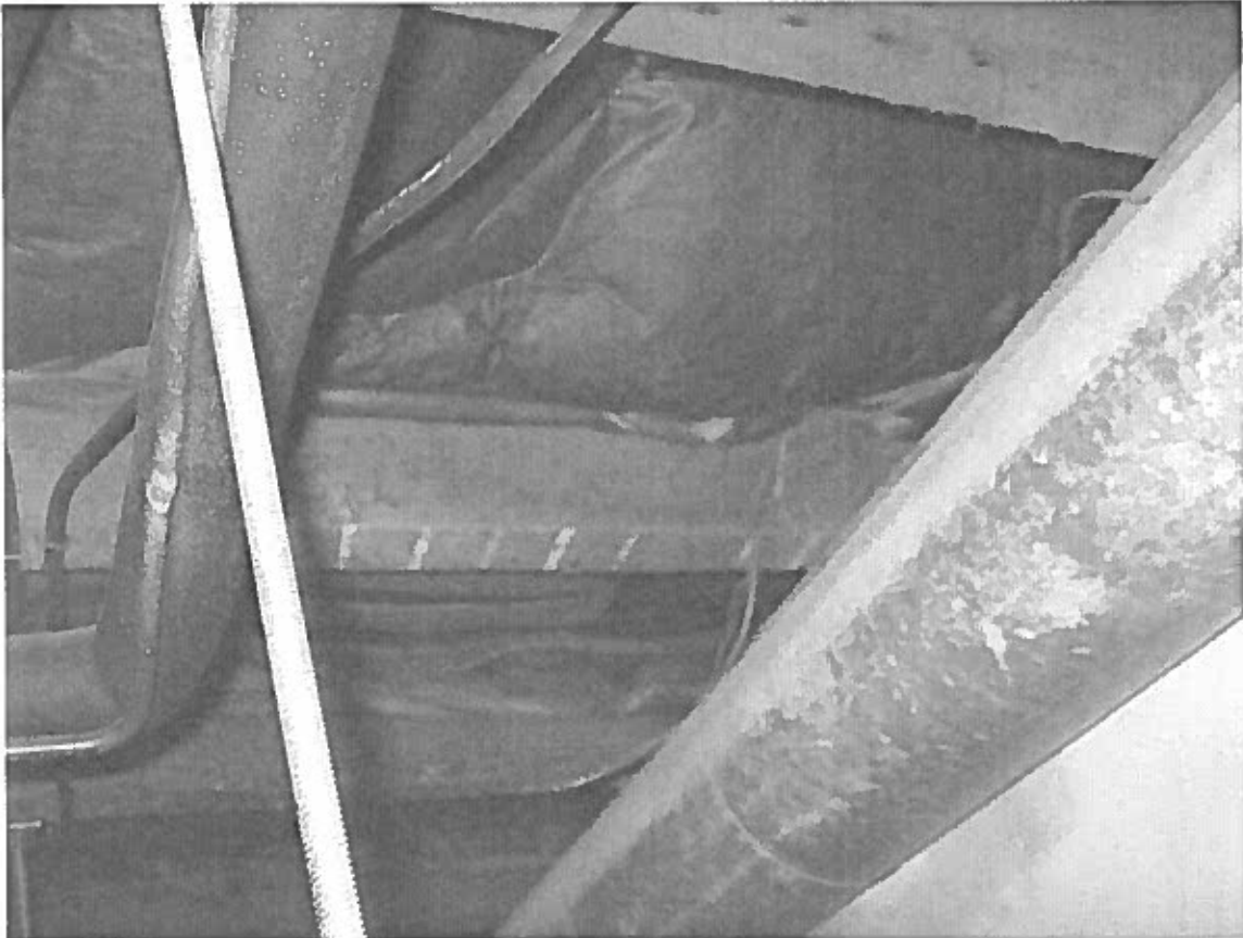
Photo 12 - Roof joists and ceiling joists 2 x 8 @ 16"
