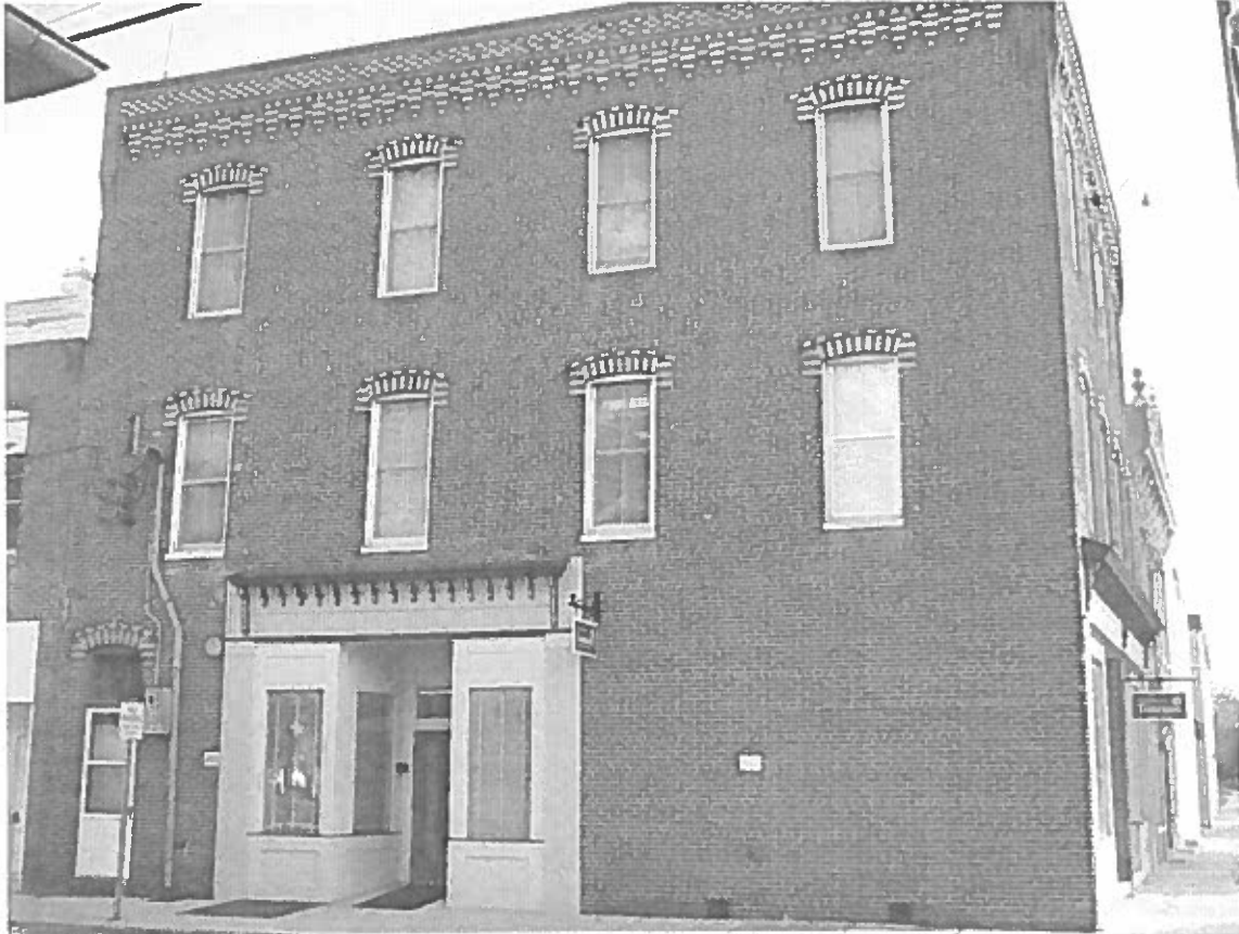
Photo 54 - Building exterior in fair condition
