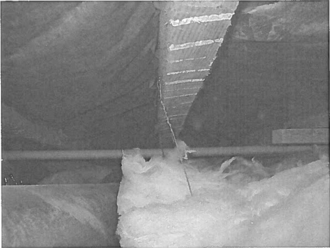
Photo 13 - Roof joists and ceiling joists 2 x 8 @ 16"
