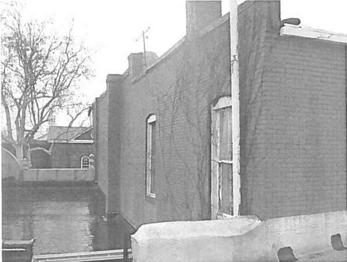
Photo 56 - Building exterior in fair condition
