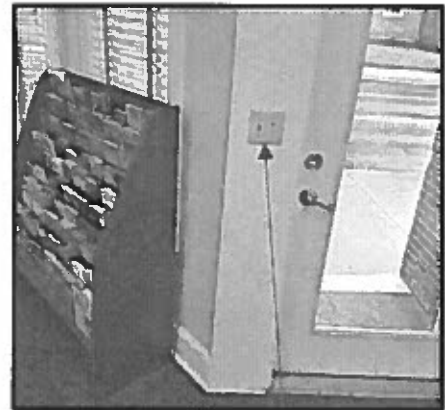
Photograph #15: Lighting Switch
