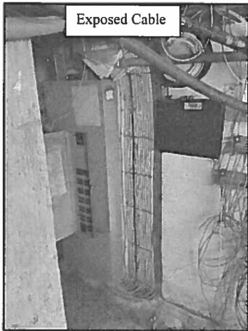
Photograph #10: Example of Non-Metallic Sheathed Cable
