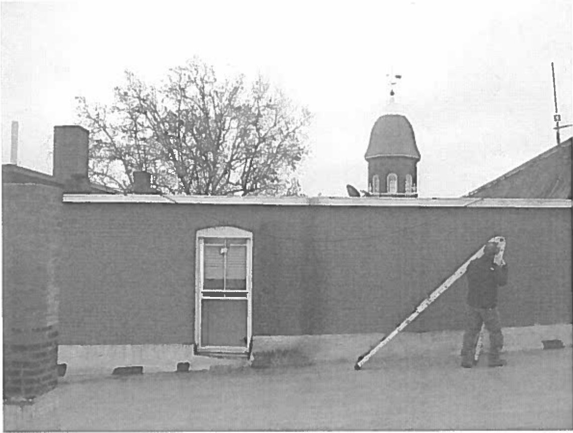
Photo 55 - Building exterior in fair condition
