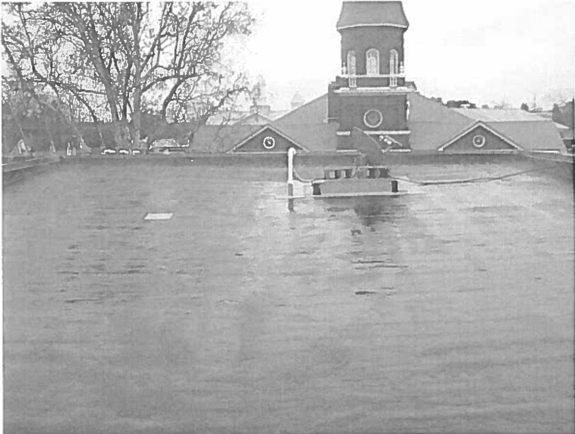
Photo 10 - Roof slope is adequate
