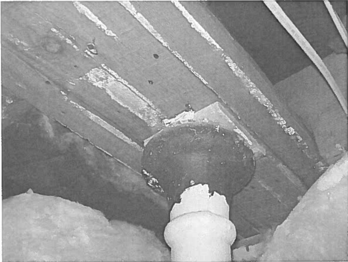
Photo 15 - Beam & column supporting roof and ceiling
