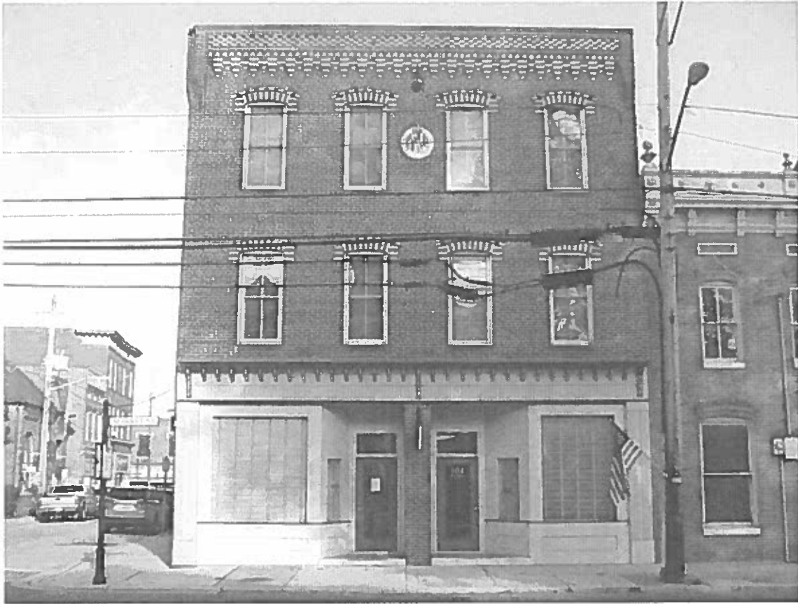
Photo 53 - Building exterior in fair condition
