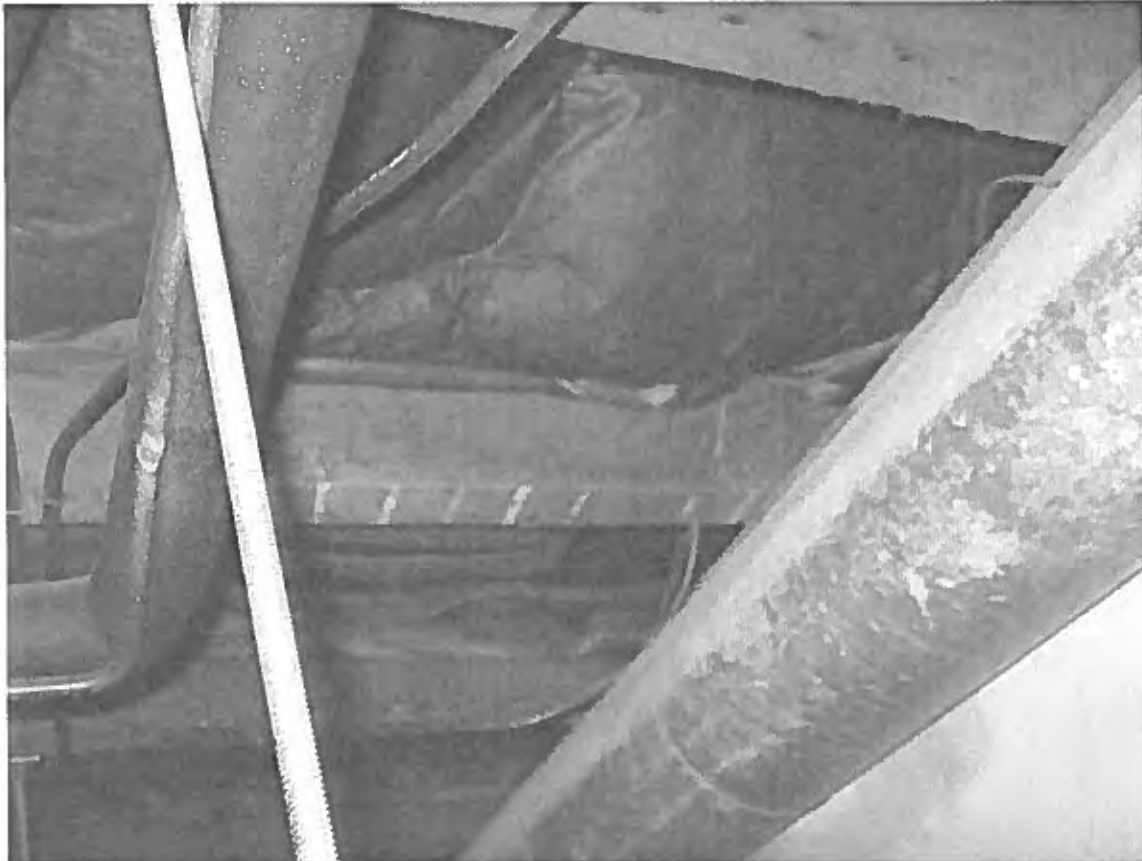
Photo 12 - Roof joists and ceiling joists 2 x 8 @ 16"
