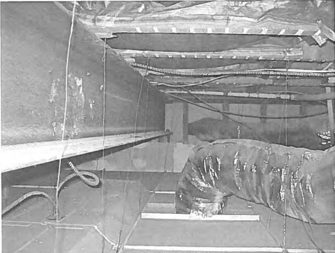
Photo 26- Supplemental support of second floor joists
