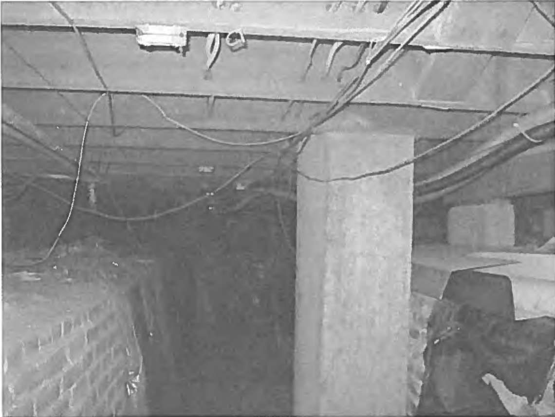
Photo 47 - Supports for supplemental framing above
