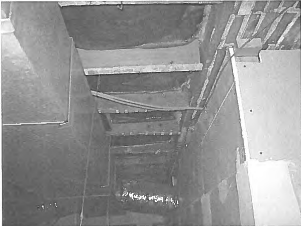
Photo 22 - Second floor framing 2 x 12 @ 16"
