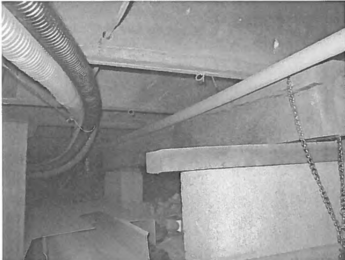
Photo 32 - Supplemental supports at joist ends
