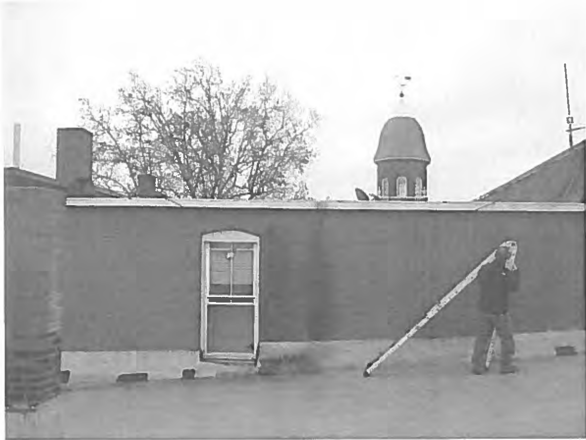
Photo 55 - Building exterior in fair condition
