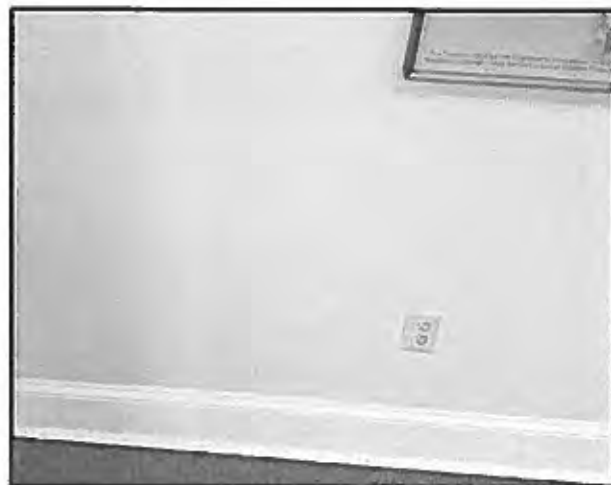
Photograph #11: Example of Receptacles (Typical Throughout Building)
