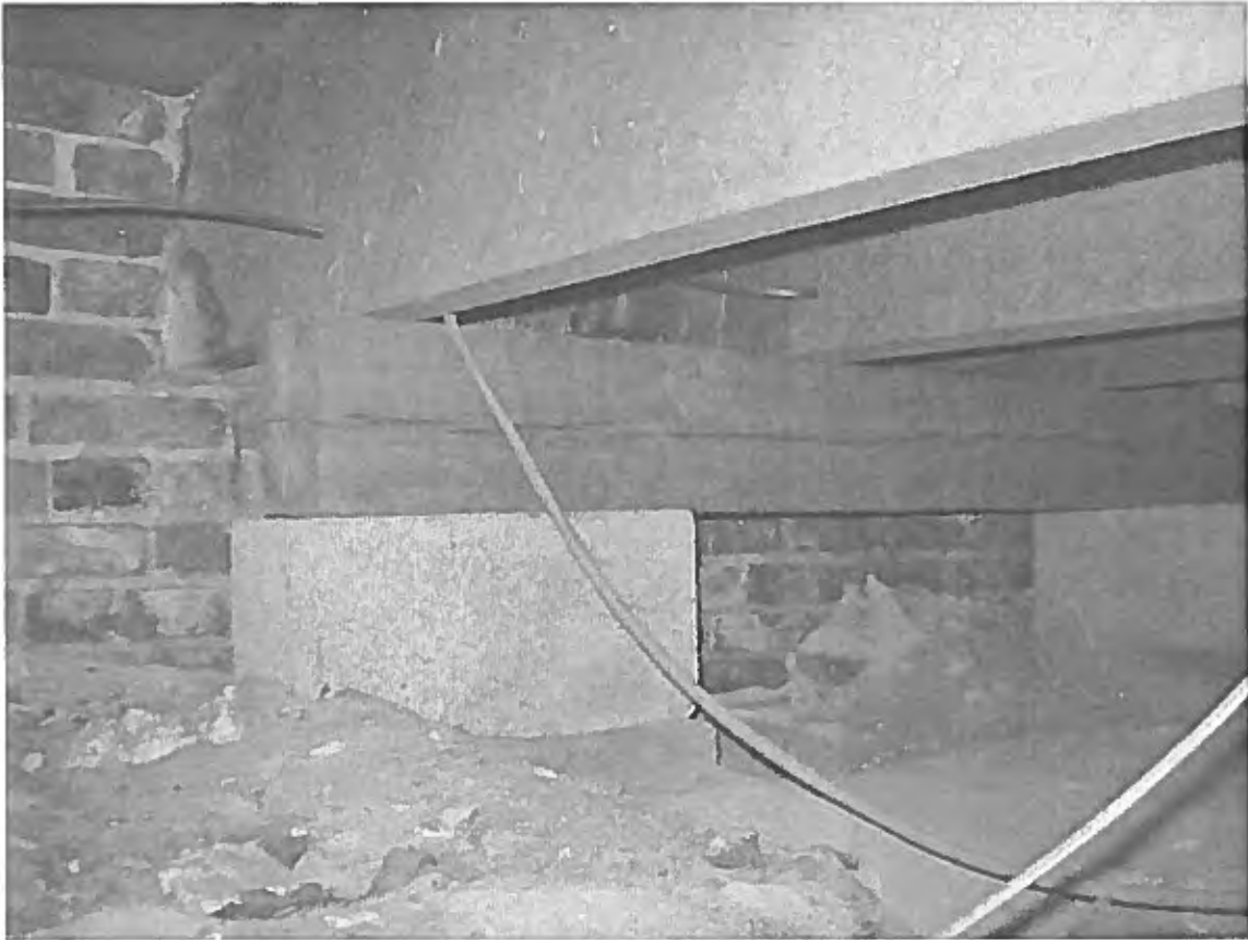
Photo 31 - - Supplemental supports at joist ends
