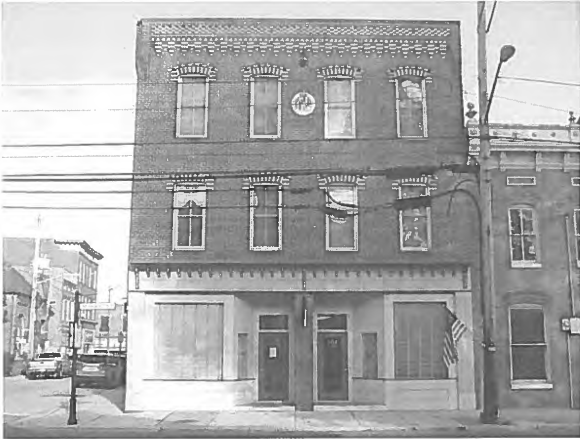
Photo 53 - Building exterior in fair condition
