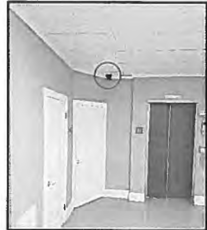
Photograph #21: Video Surveillance Camera
