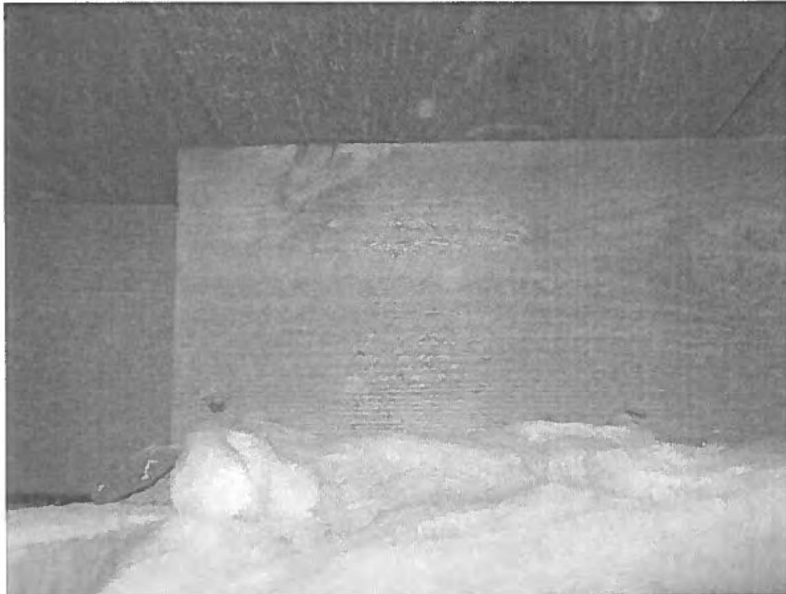
Photo 14 - Roof joists and ceiling joists 2 x 8 @ 16"
