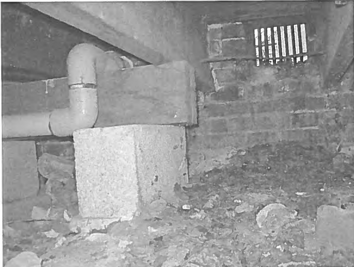
Photo 30 - Supplemental supports at joist ends
