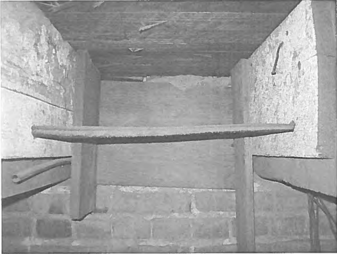
Photo 45 - Steel columns above bear on interior wall
