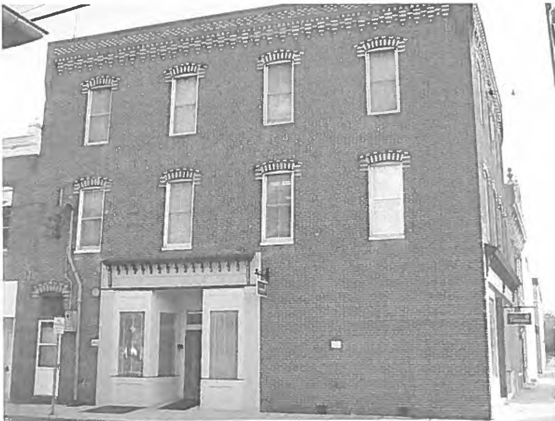
Photo 54 - Building exterior in fair condition
