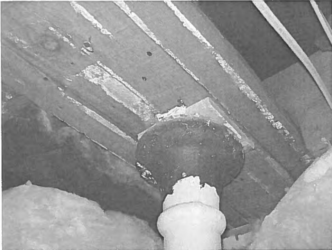
Photo 15 - Beam & column supporting roof and ceiling
