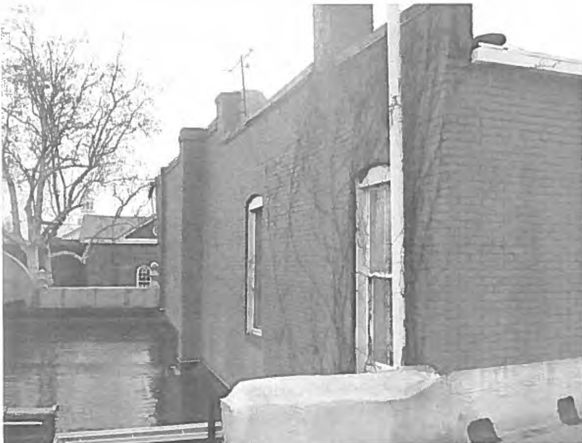
Photo 56 - Building exterior in fair condition
