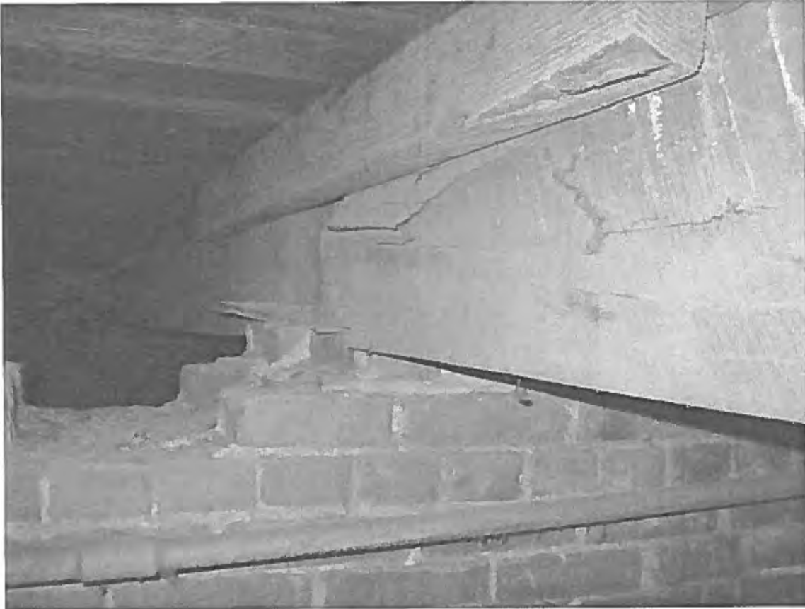
Photo 29 - Joists bear directly on brick walls
