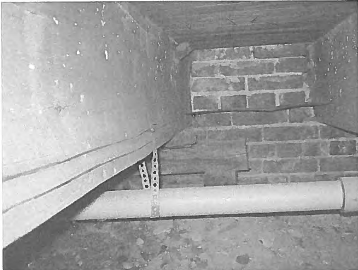
Photo 28 - First floor framing 2 x 12 @ 16"
