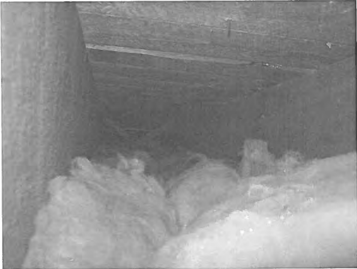
Photo 19 - Third floor framing 2 x 12 @ 16"
