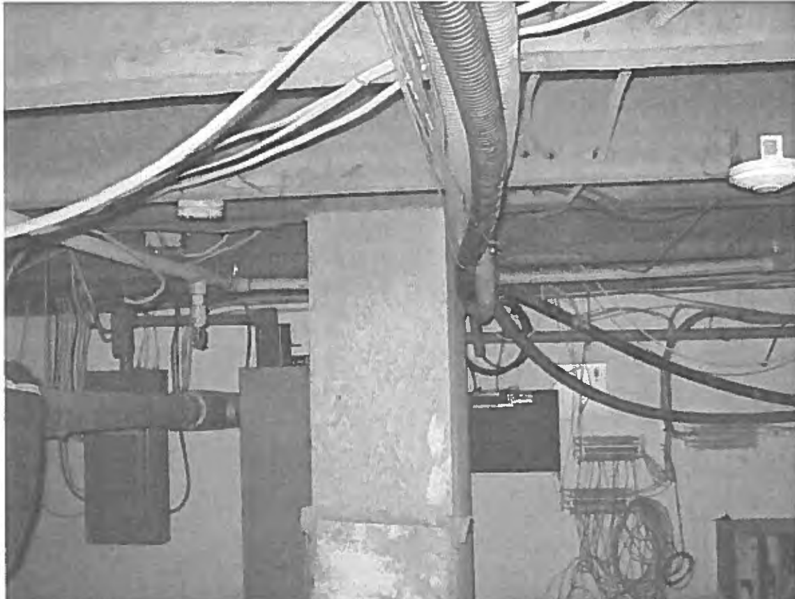
Photo 48 - Supports for supplemental framing above
