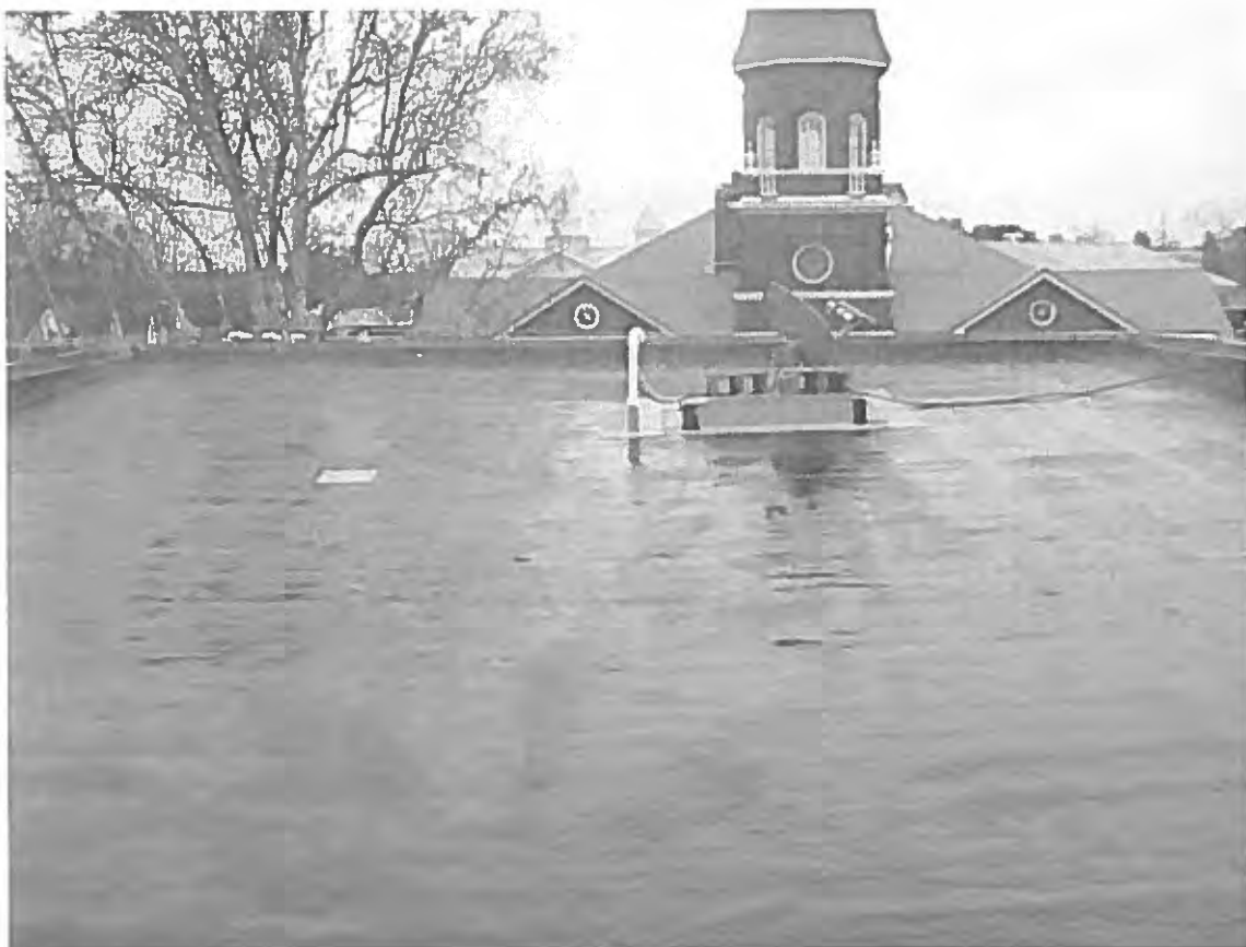
Photo 10 - Roof slope is adequate
