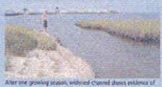
After one growing season, widened channel shows evidence of scouring by tidal action, which prevents buildup of sand. Biodegradable bags behind with wooden stakes and cause after removal of metal bars.
