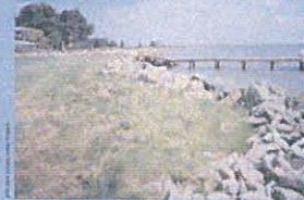
Riprap built with piled rocks.
