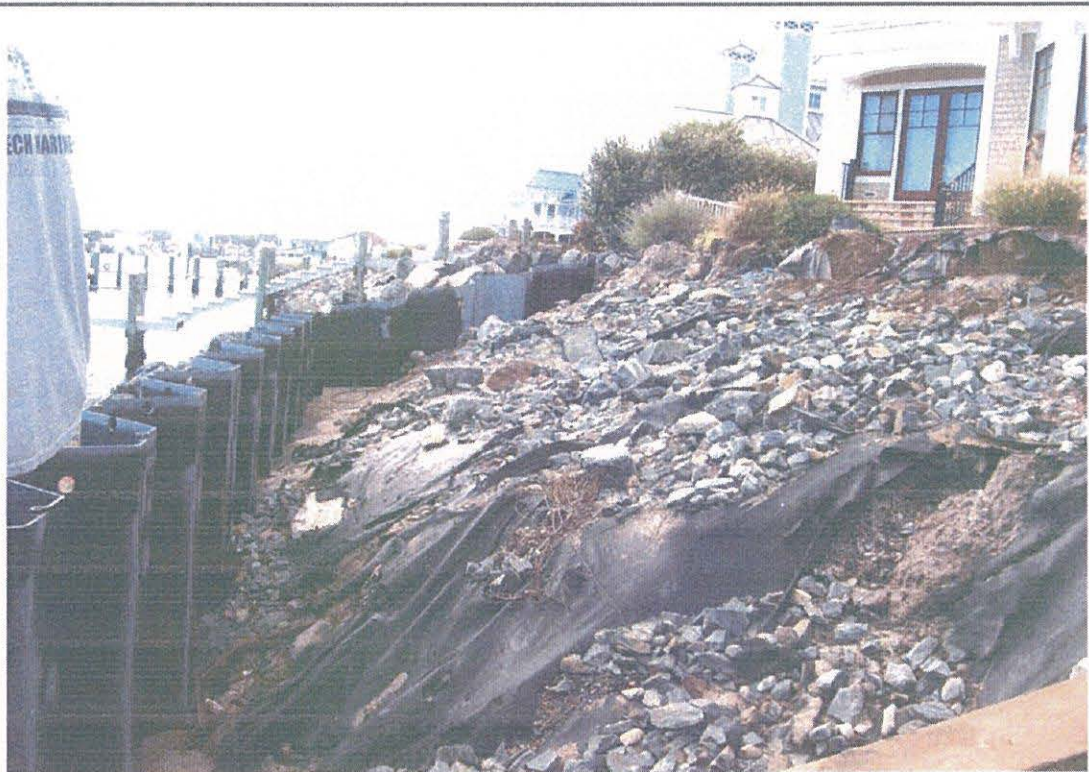
CONSTRUCTION: Photo showing the steel bulkhead installed above MHW
