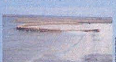
Marsh bed created with coarse sand fill double-staked bivalve back the-groin sills.
