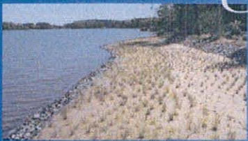
Living shorelines help protect the shoreline from erosion. Photo by John C. Silliman, University of Maryland System.
