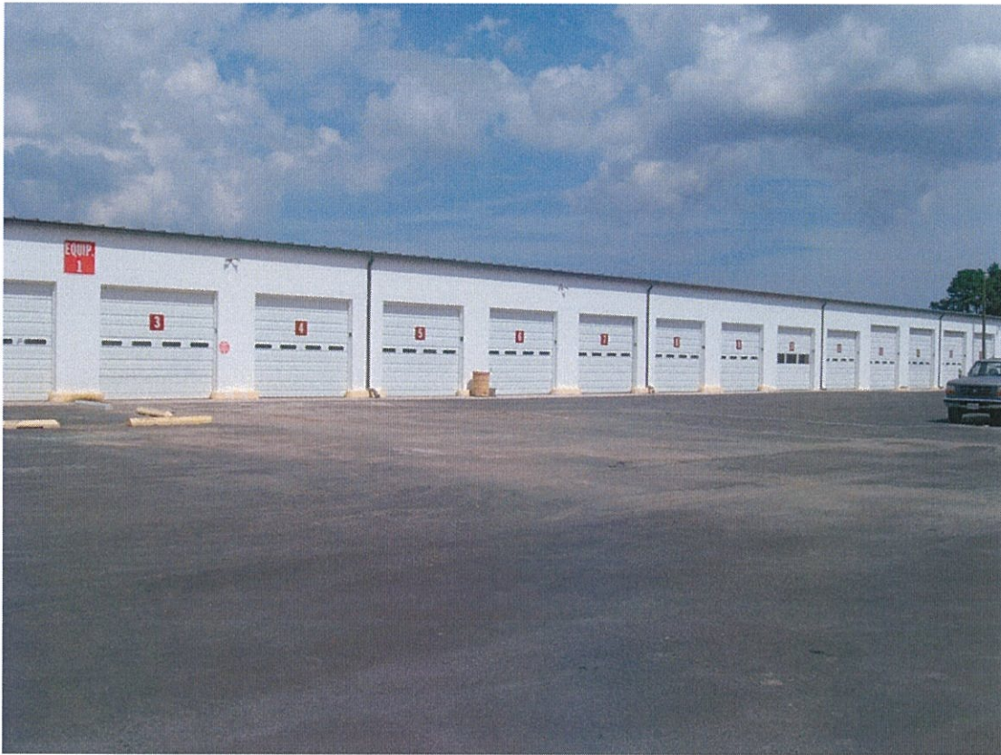
Enlarge and Replace Doors 3 thru 11 – 5764 Worcester Highway – DPW Roads Divison
